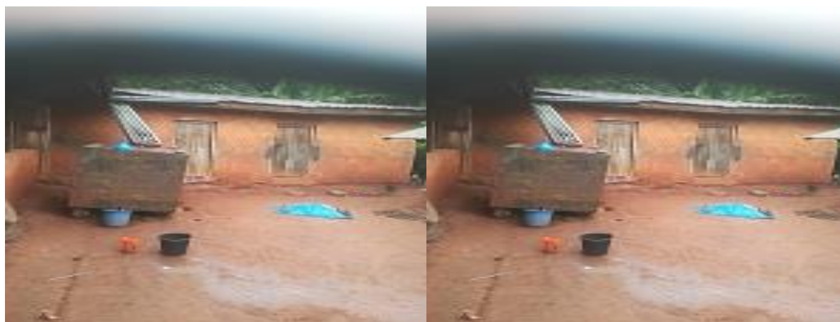
Fig. 2: Water storage facilities.
